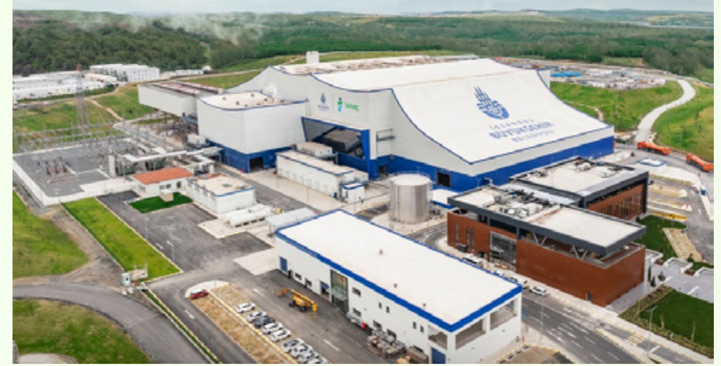
Figure 12. Municipal Waste Incineration Facility of İstanbul Municipality
